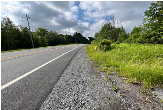
FACING SOUTH ALONG RT 42
